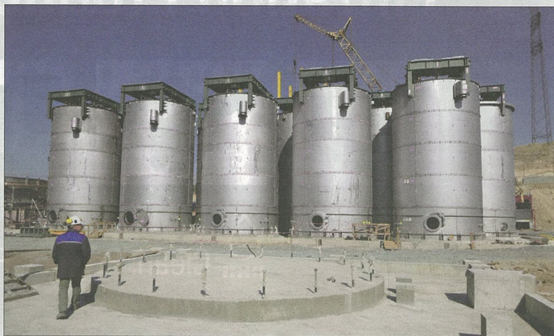
Robust: The bolted and modular ZipaTank suits the robust requirements needed to store abrasive slurries.
