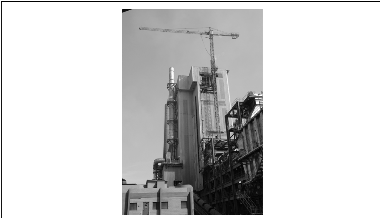
Figure 8: SPCC Ilo Smelter Copper ISASMELT™ plant view
