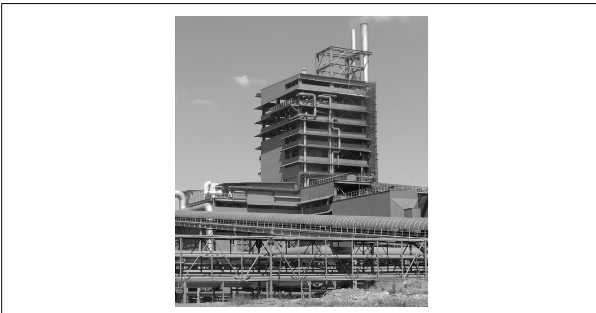
Figure 5: View of the YCC Chambishi ISASMELT™ Plant in Zambia
