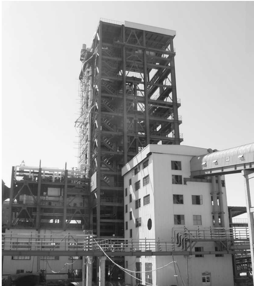
Figure 4 - The ISASMELT building during construction
