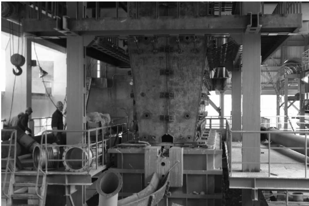
Figure 5 - YMG Blast Furnace during construction.
